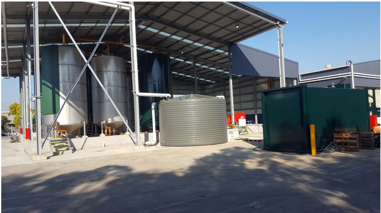
Used oil tank farm within roofed bunded area (not commissioned). Rainwater tank for collection of roof water.
