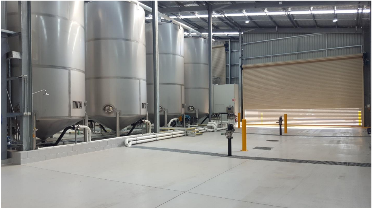
Sludge and aggregated Food Waste storage tanks and dispatch loading bay area.
