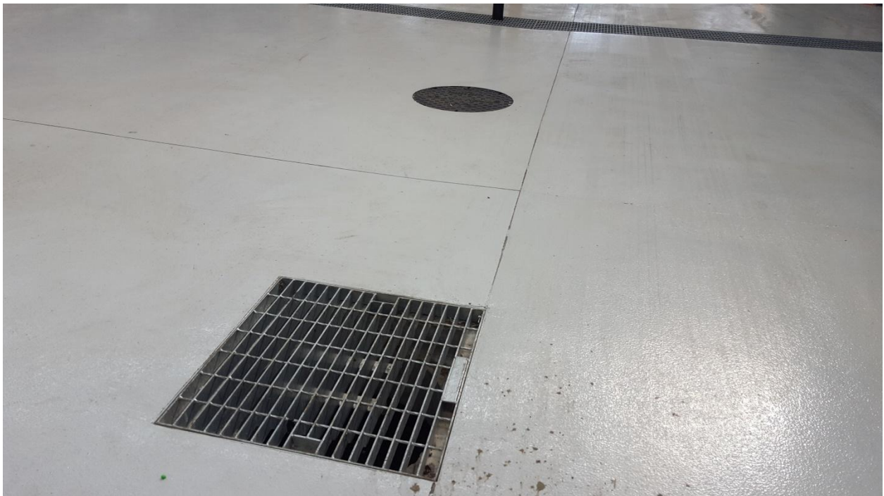
Imperviously sealed floor with in-ground sump for spill containment.
