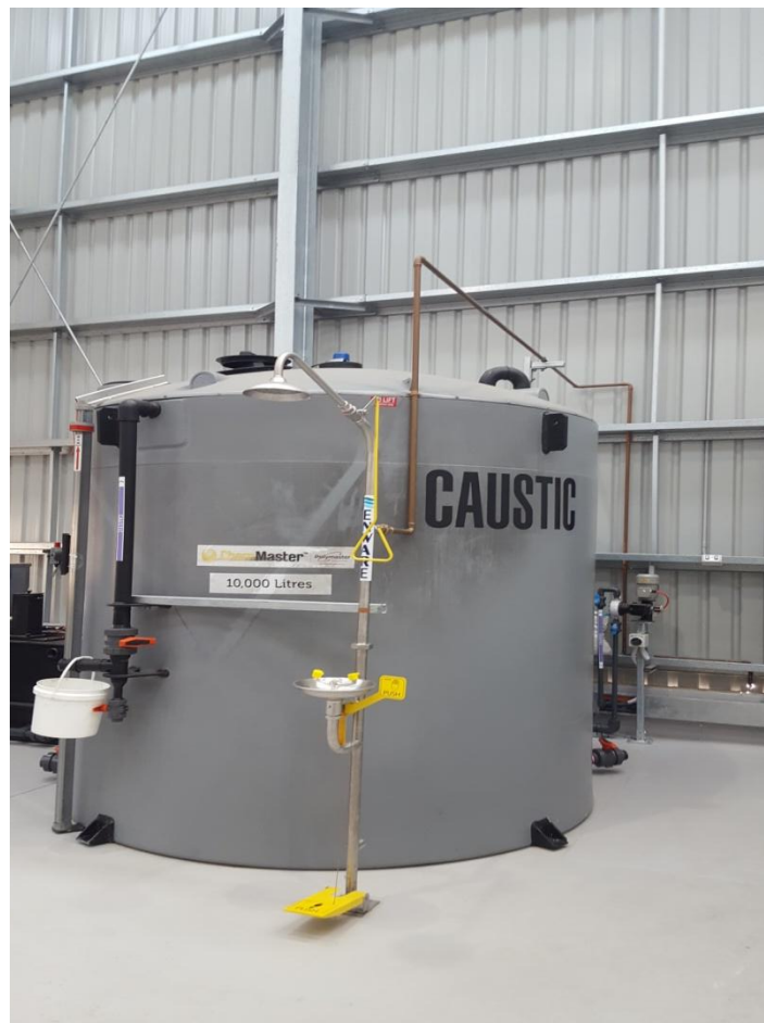
Caustic stored within the bunded tank farm area & used to adjust the pH within the DAF Unit
