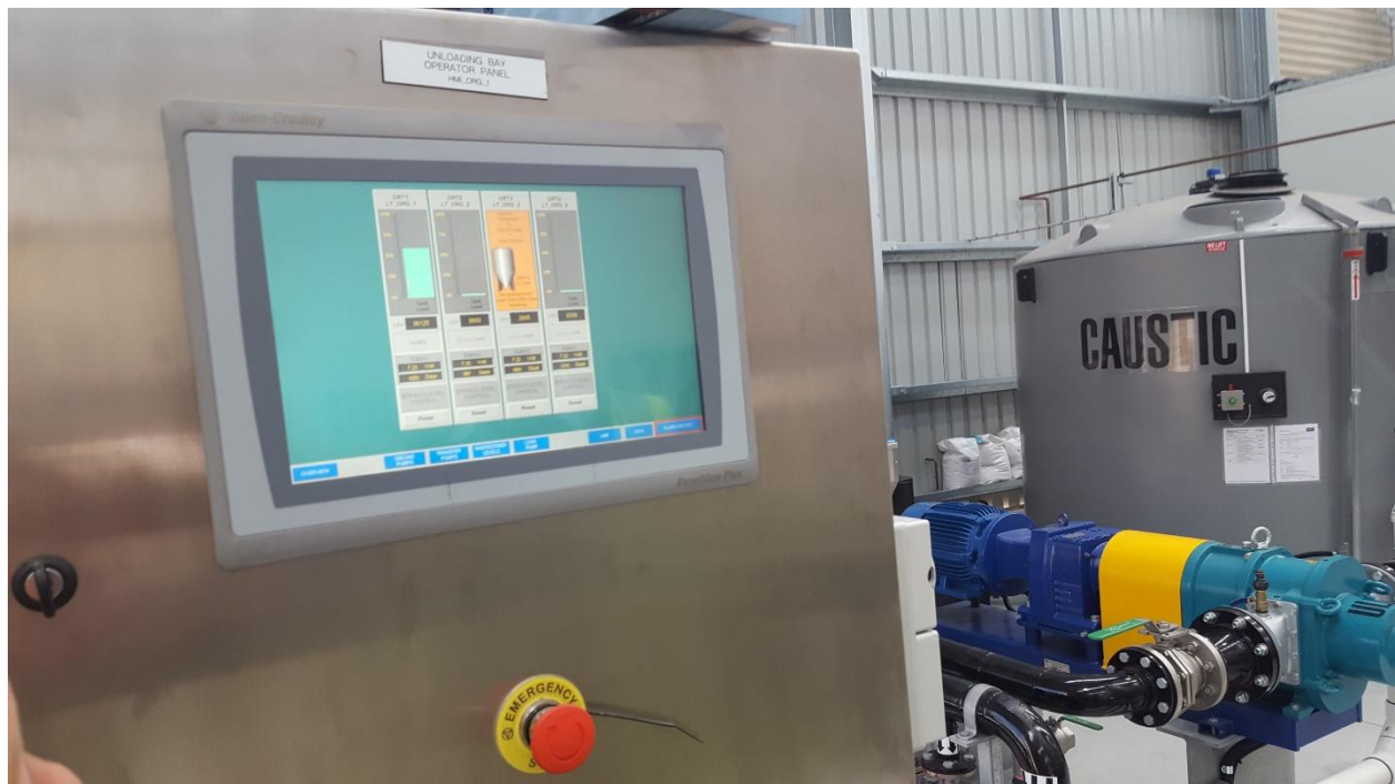
Incoming organic waste unloading bay monitoring system and emergency stop button.
