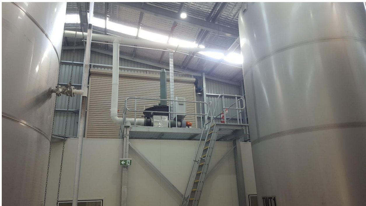
Odour Control Unit located above the DAF unit enclosed room.
