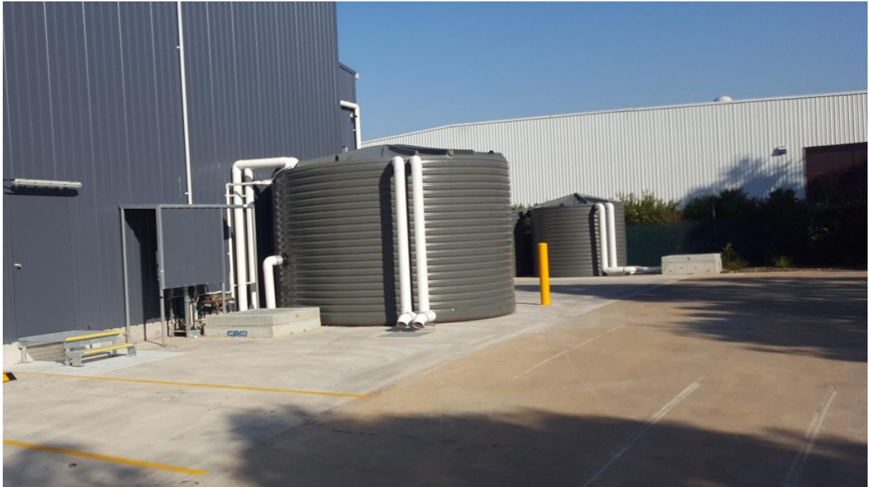
Rear of Organics Building – Rainwater tanks and SPEL stormwater infrastructure observed to be in place.
