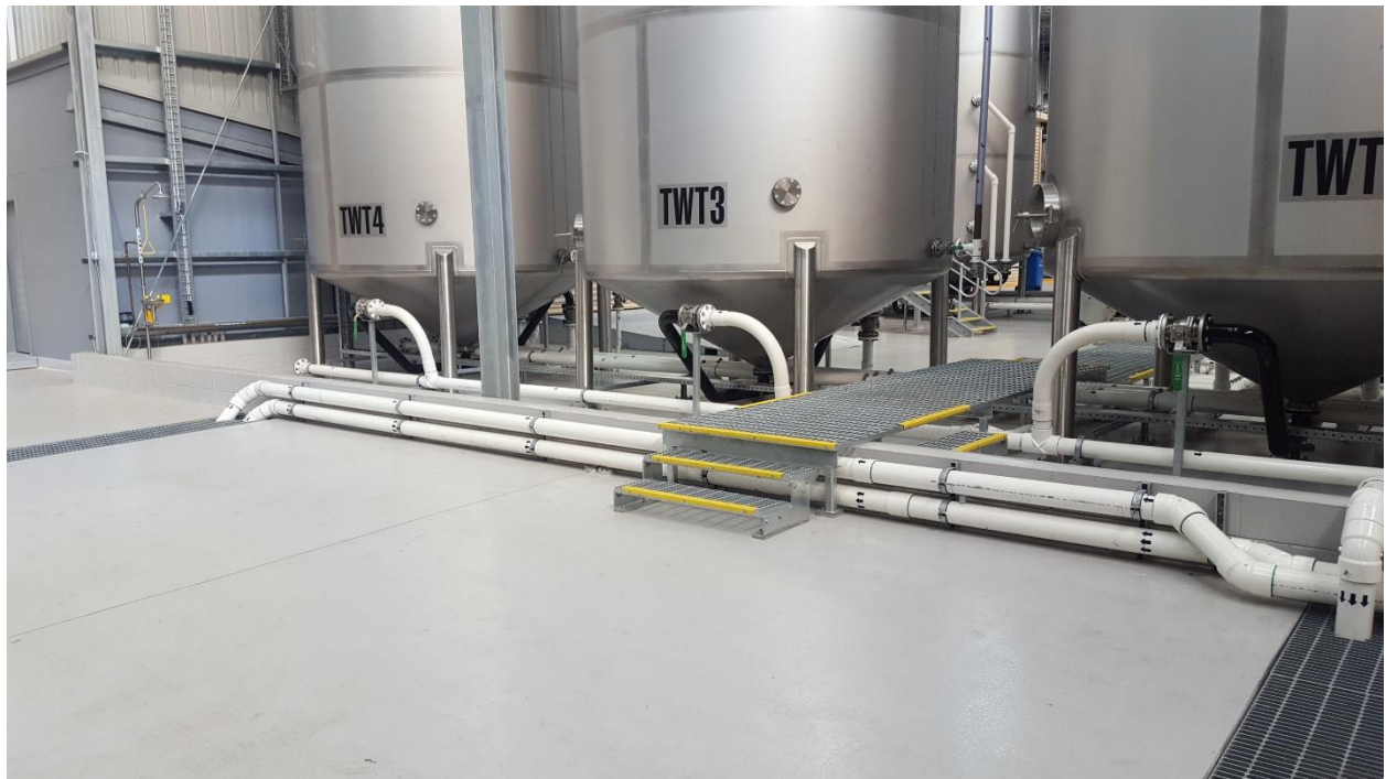
Pipework going over bund walls
