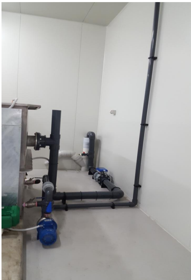
Trade Waste connection within DAF Unit room.
