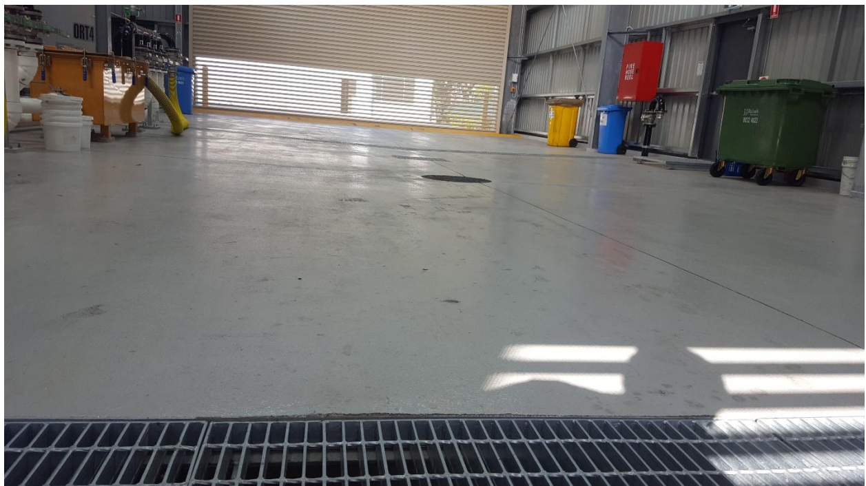
Bunded incoming organic waste unloading area drive-over bunding and in-ground sumps for containment of waste material.
