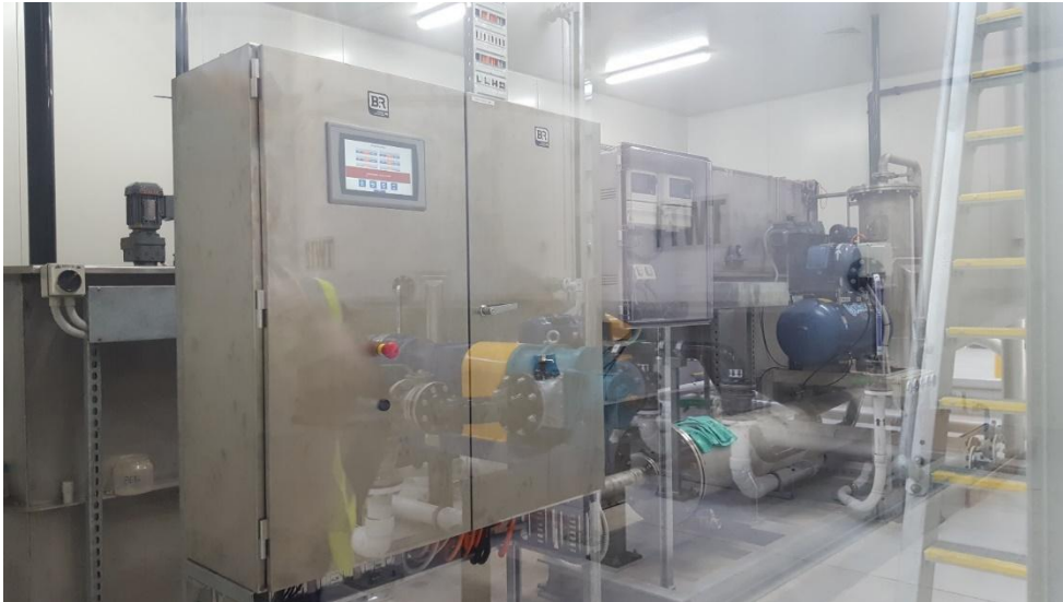
Dissolved Air Flotation (DAF) Unit within enclosed room.
