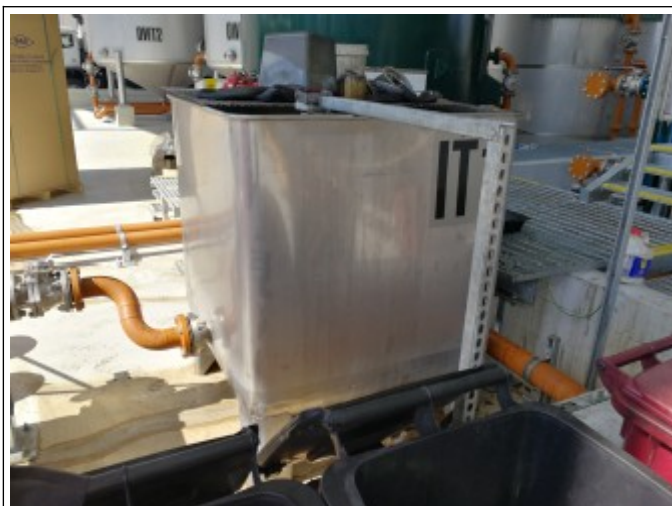
Short-term oily water transfer container
