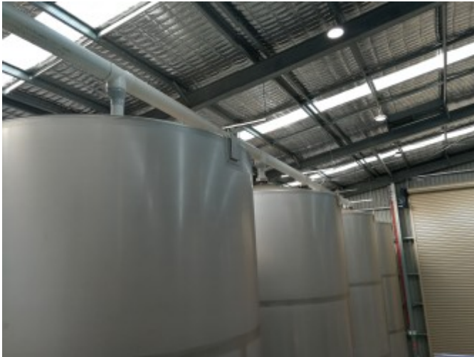
Ducting above sealed organic waste tanks connected to OCU
