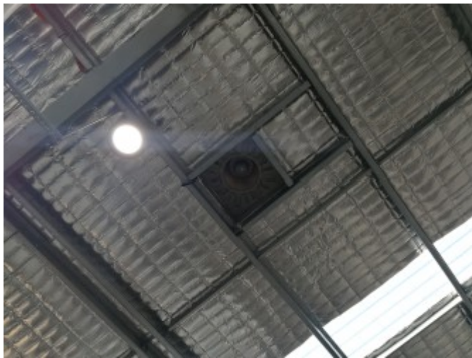
1 of 8 rooftop mechanical exhaust fans (nearest to OCU outlet)
