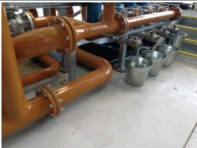
Collection trays below oil filters
