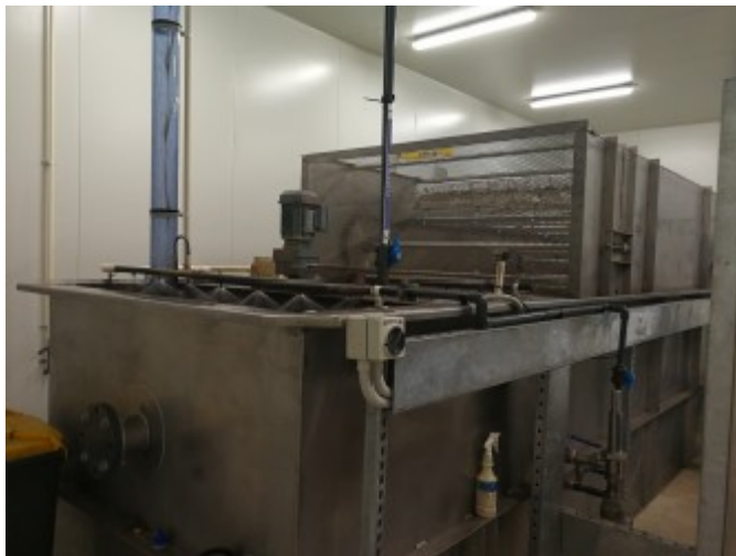
DAF unit inside enclosed room
