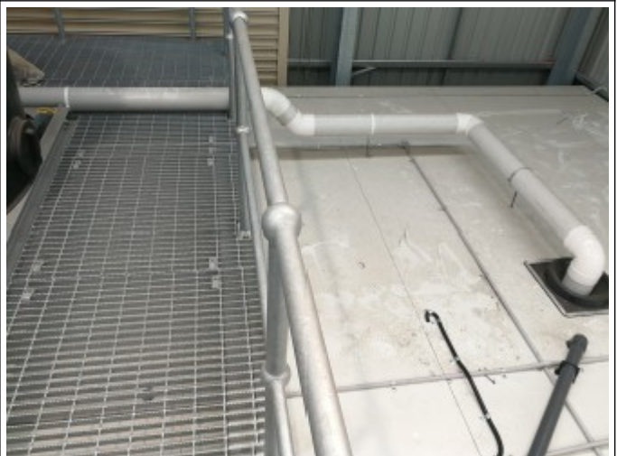
Roof of DAF building – second ceiling vent connected directly to odour control unit ducting
