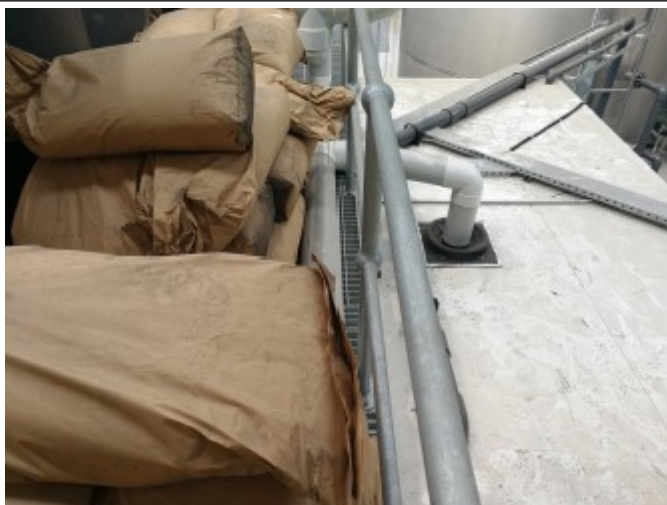
Roof of DAF building – ceiling vent connect directly to odour control unit ducting
