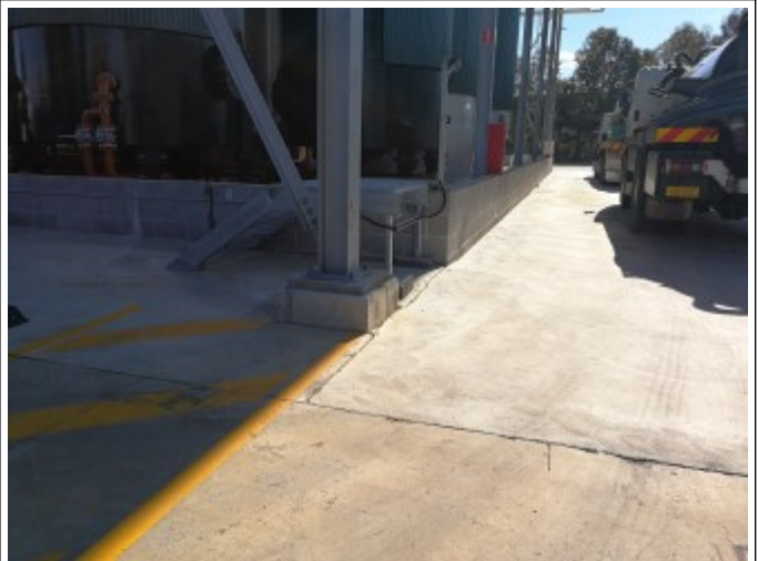
Bunding around waste oil tanks
