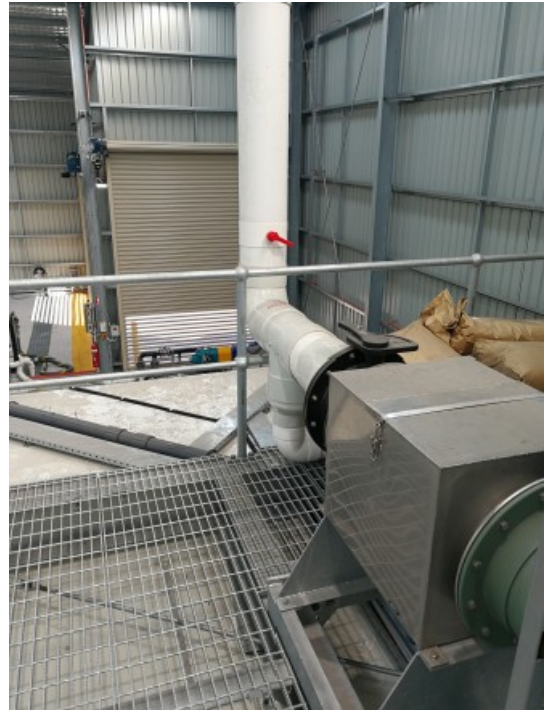
All tank ducts combine to a single point which passes through the OCU
