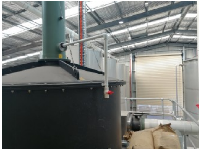
Sampling port to OCU outlet with extended ducting for qualitative observations
