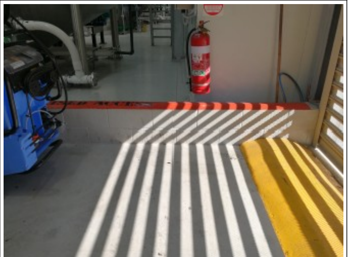
Bunding separating unloading area from organic tanks
